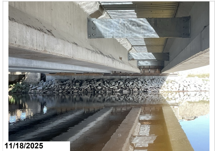
Bent 1: integral abutment overview.
