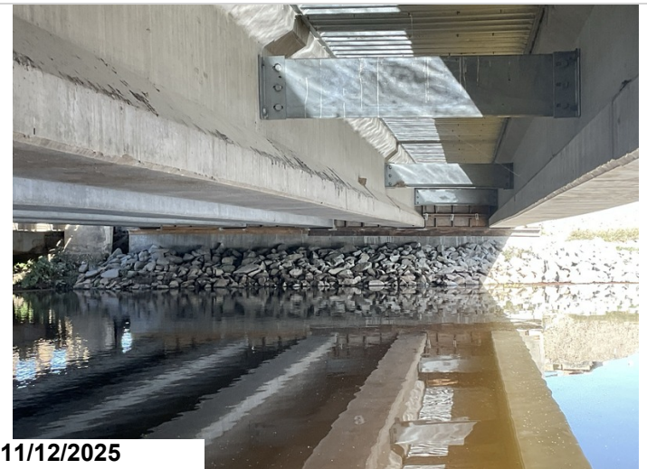
Bent 1: integral abutment overview.
