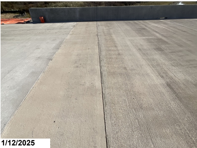
Bent 1, joint seal: general pourable joint seal condition.
