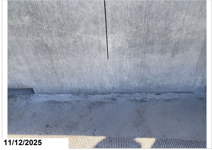
Left rail: cracking measuring 0.012" at each saw cut relief. CS2-6'
