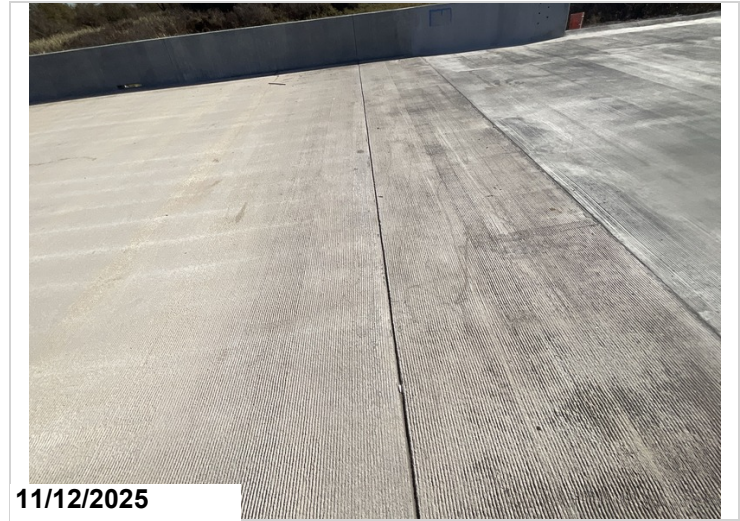
Bent 2, joint seal: general pourable joint seal condition.
