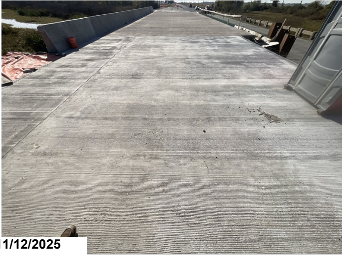
Bent 1, approach slab: general approach slab condition. (North approach slab)
