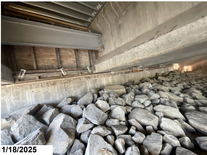
Bent 2: integral abutment overview.
